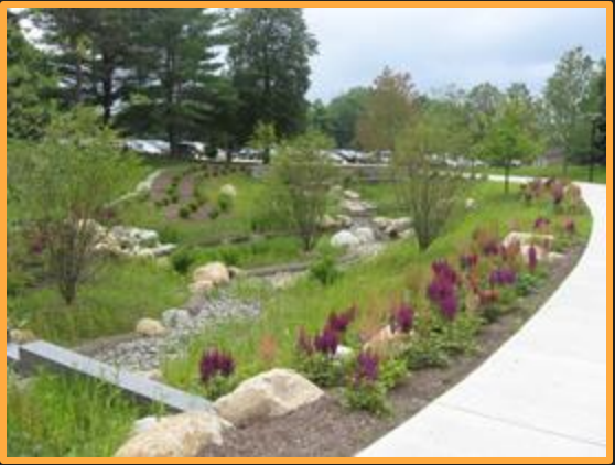
Rain Gardens and Bioretention
