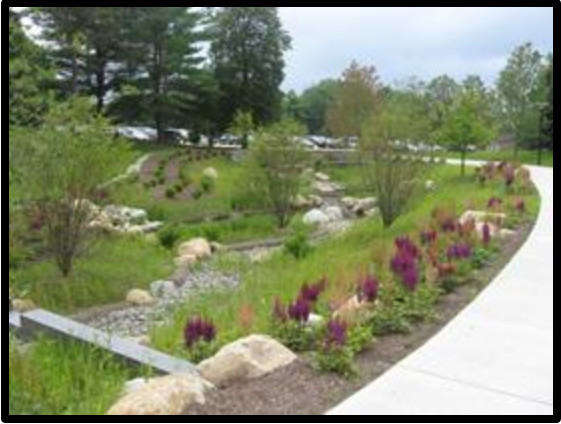
Rain Gardens and Bioretention
