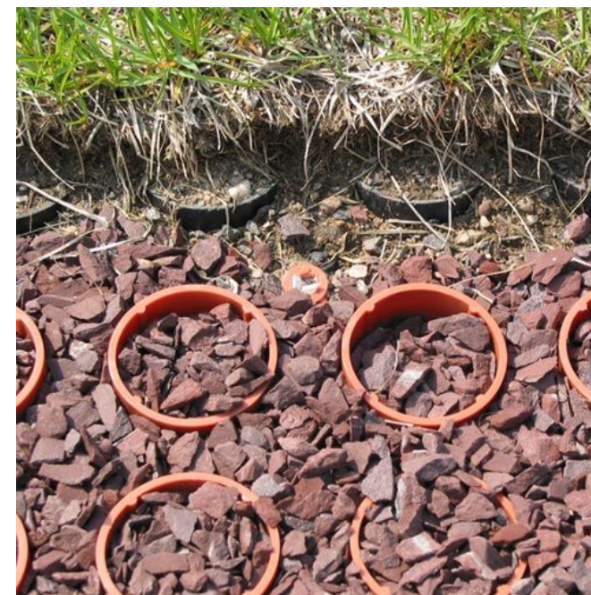
Gravel Grid Pavement
