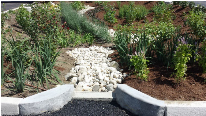
Figure 13-39. Typical Inlet Curb Cut Openings
