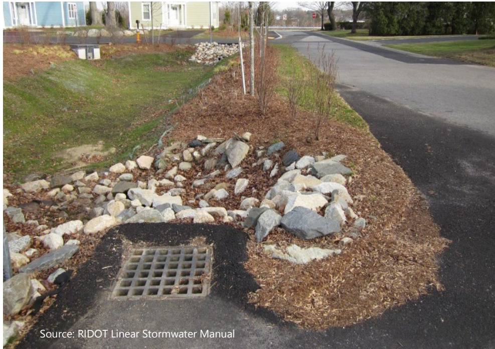
Figure 13-40. Deep Sump Catch Basin Inlet Structure
