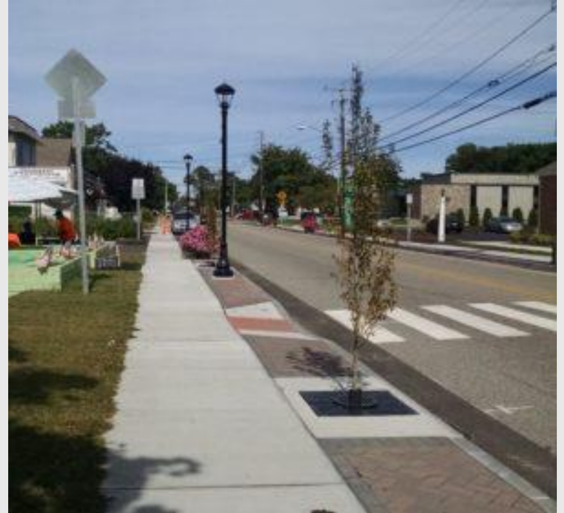
Tree filters in downtown Niantic, CT
