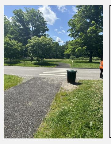
Irwin Park already has several pervious pavement paths, specifically made of a material called Flexi-Pave. The photo on the right shows a path made of Flexi-Pave that would lie right next to the potential rain garden. Having both green stormwater practices work in tandem could prove very beneficial for both the surrounding environment and educational benefits towards the community. This serves as an opportunity to further provide education to the community.
